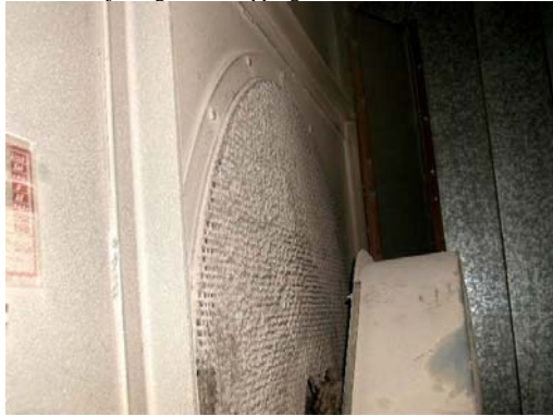
2m dia Richardson RA Fan classed as a Fire Fan
